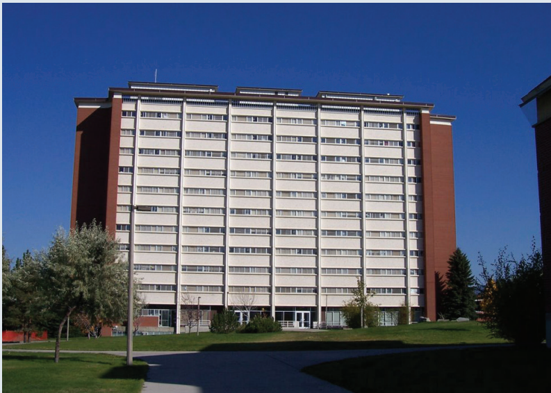
North Hedges Hall, Montana State University; Bozeman, Montana
