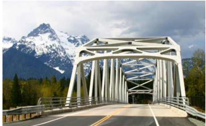
Sauk River Bridge photo courtesy BergerABAM
