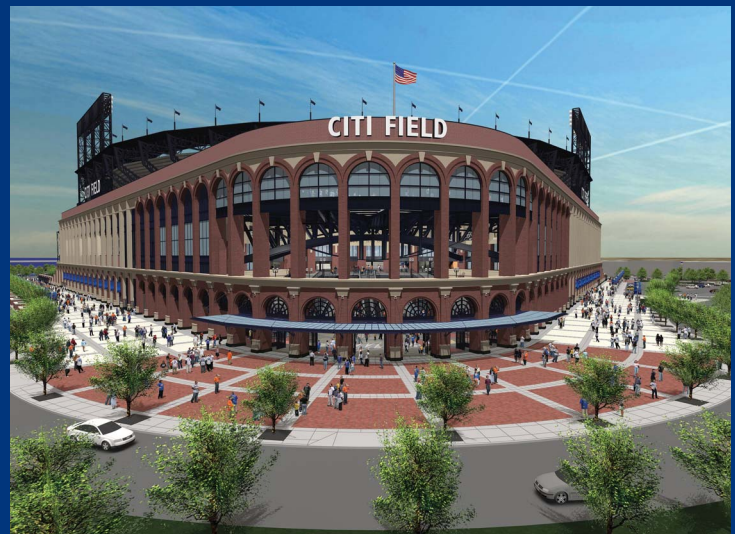
Team members on the Mets' Citi Field ballpark project are using Newforma Project Center software to streamline key components of their process.
